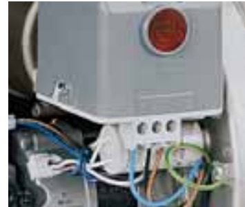
Control box fitted with an ignition transformer
