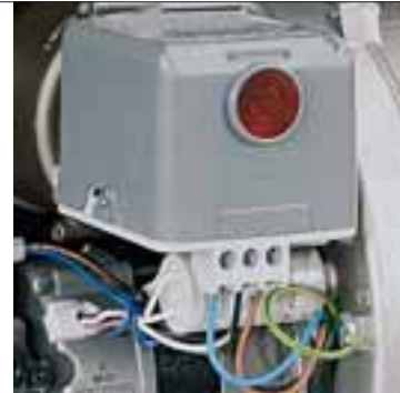
Control box fitted with an ignition transformer
